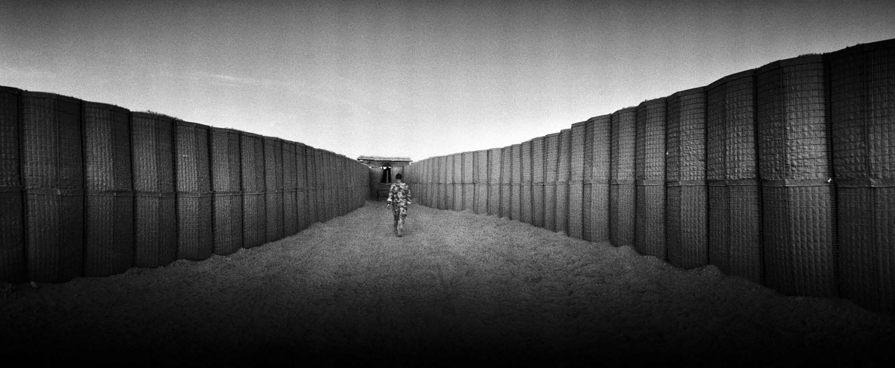
Bagram, Afghanistan 2007. Freshly fabricated sections of concrete blast walls outside Bagram airbase.
